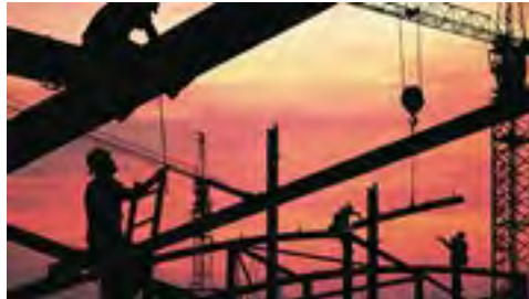
House Budget Committee Chairman John Yarmuth (D-KY) is developing legislation that would create a National Infrastructure Development Bank, which would be financed through the sale of $75 billion worth of Rebuild America Bonds on the full faith and credit of the U.S.
